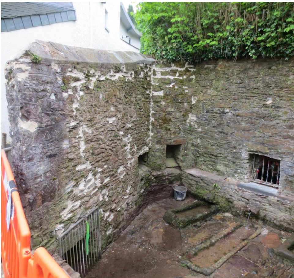
Fig.5 Caught just in time? Substantial repairs were needed to the left hand wall, probably the most recently built element of the well.
