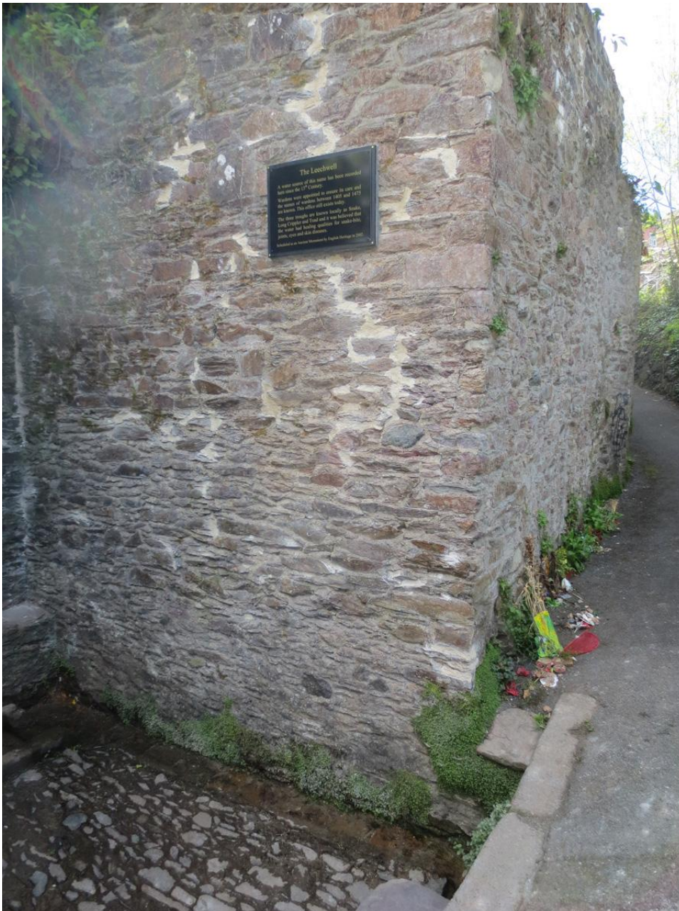
Fig.6 The board is unobtrusive but legible from below, the text can be found in Section 6. Hopefully, the board will be out of reach of graffiti artists. Some large cracks in the wall have been repaired. A depressed channel drains water along the base of the wall from the trough called 'Toad'.
