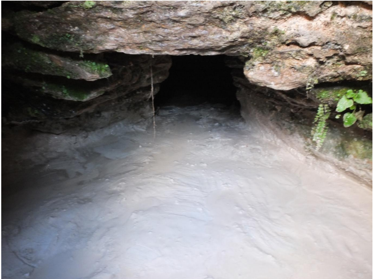
Fig.15 Newly re-puddled interior complete.
