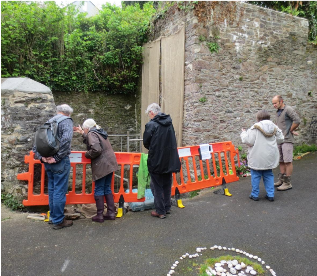
Fig.3 Meeting at the well. Left to right: James Bellchambers, Shirley Prendergast, David Martin, Pruw Boswell, Bruce Kirby. Dave Mitchell is taking the photograph. (The hessian protecting the new lime mortar is still in place)
