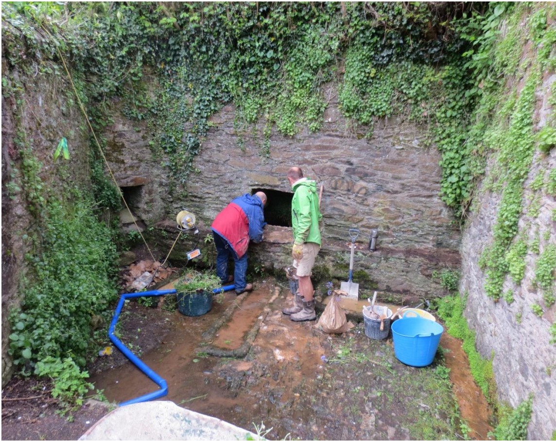
Fig.2 The well overgrown and neglected. Bruce and Will remove the old red clay base.
