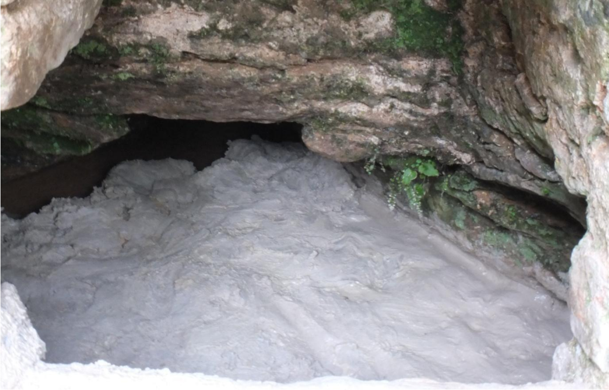
Fig.13 Working backwards towards the neck and channel with the clay. The shallow opening to the inner chamber can be clearly seen. The interior is in good condition, only a few small repairs were needed.
