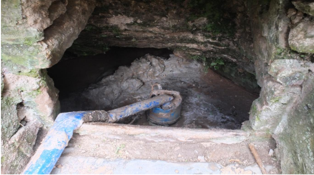
Fig.11 A dam was formed and a pump was used to remove as much water as possible.
